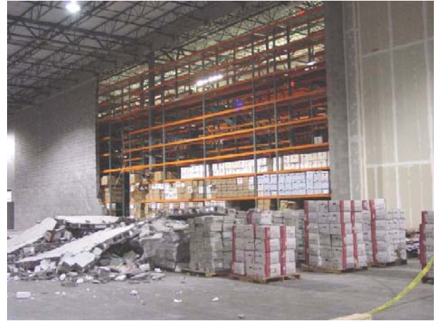
Fig. 5: An example of a high pressurization of the enclosure volume.
