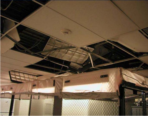
Fig. 3: An example of a high pressurization of the enclosure volume (false ceiling)
