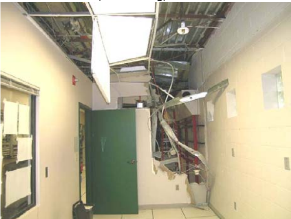
Fig. 4: An example of a high pressurization of the enclosure volume.
